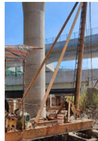
应力消散孔施工
