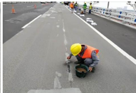
裂缝灌缝
